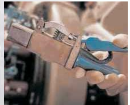
If caution is exercised during removal of the plug-in brush holder, the risk of unintentional contact with current carrying or rotating machine components can be as good as eliminated.
